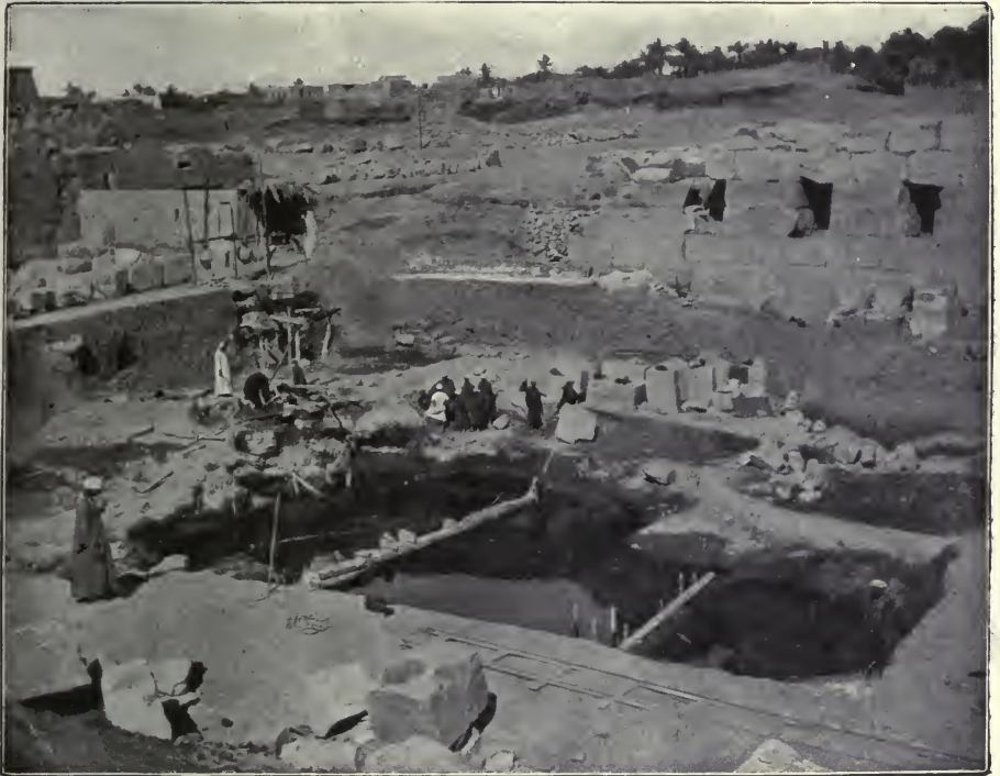
THE WORKS AT KARNAK IN JANUARY, 1906.
