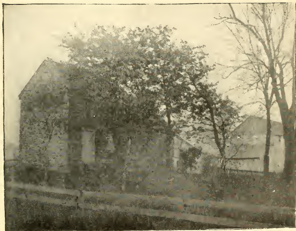
ISAIAH DEWEES' HOUSE, HOLMESBURG
