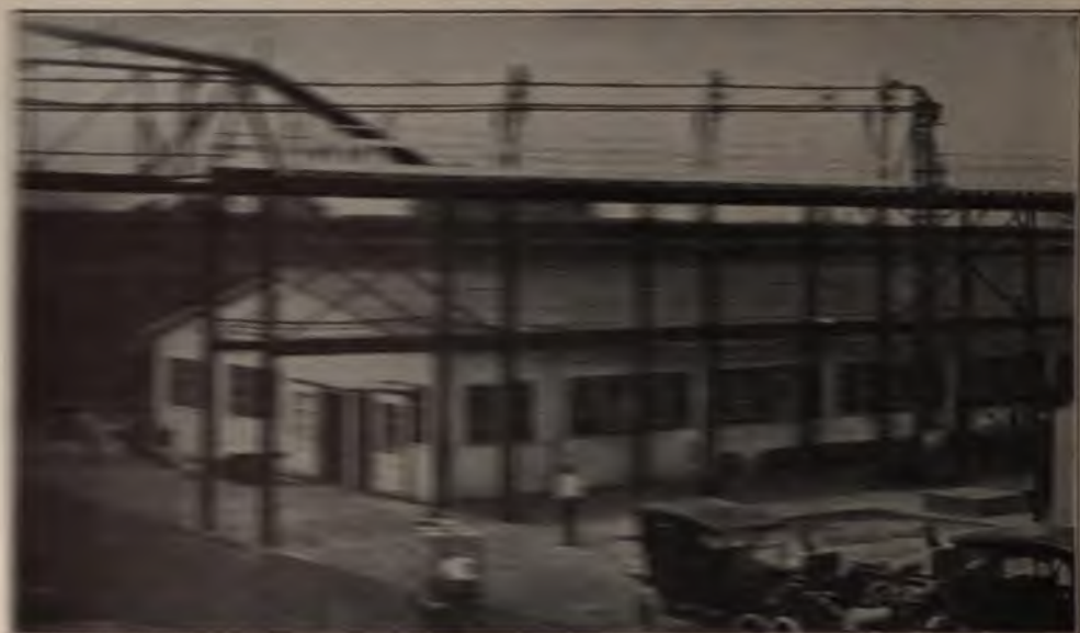
Aerial Railway Down which the Wheels Travel to the Paint Shop See pages 125 and 127
