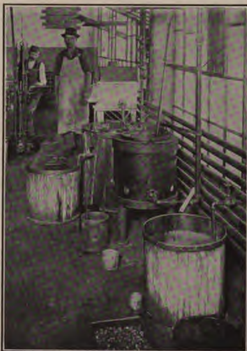
Roller and Roller-Pin Hardening and Tempering Plant; Ford Construction
