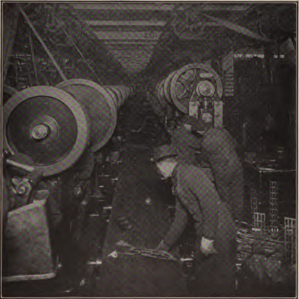
Endless Belt Conveyor between Two Rows of Punch Presses
