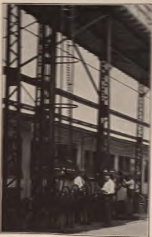
Elevator Lifting Wheels to Start Them on the Journey along the Aerial Track to the Paint Shop
