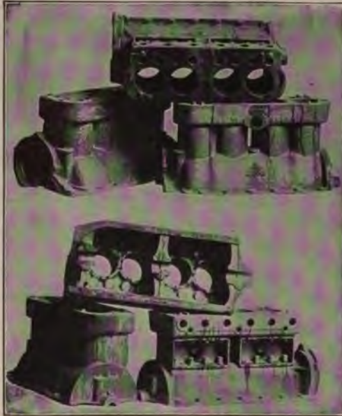
Six Views of the Ford en bloc Cylinder Casting
