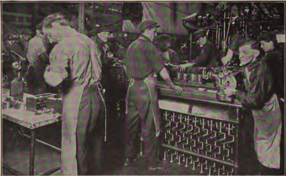
Operations 29 to 34, Inclusive—Beginning of Second Assembly Line; Placing the Crank Shafts
