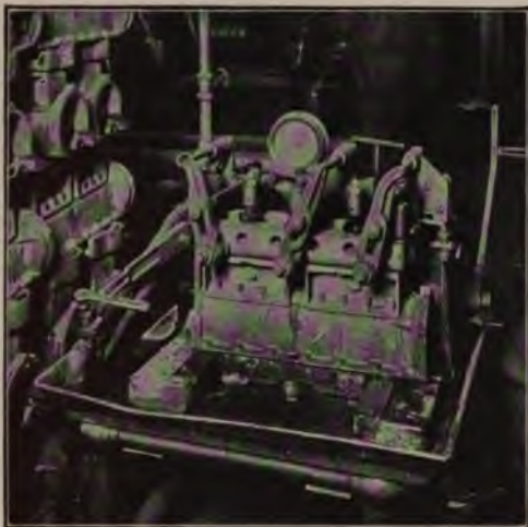
Operation 6. Hydraulic Test for Possible Leaks in Water Jacket Ford machine, design and construction
