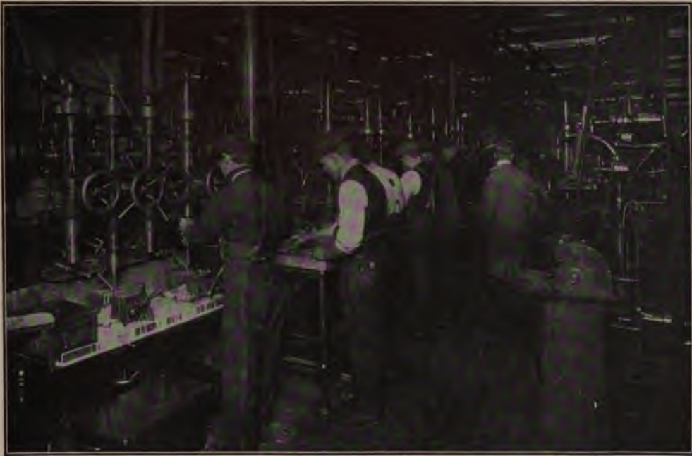
Illustrating the Close Placing of Machine Tools in the Ford Machine Shop
