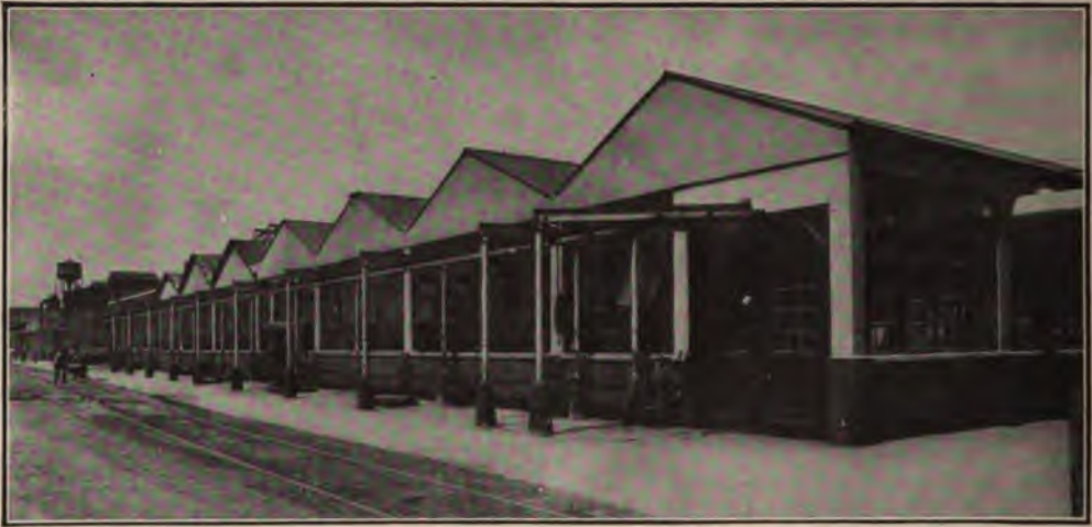
Ford Foundry, South Side from East End, Showing Overhead Monorail
