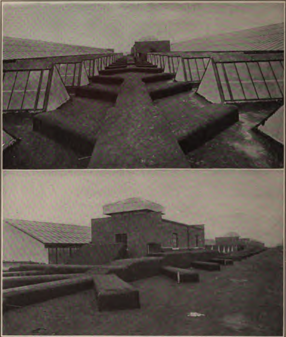
Roof of the North Buildings Showing Skylights, Air Ducts, Pent Houses, and Crane-way Glass Roof
