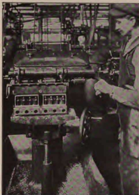
Filleting Crank-Shaft Bearings
