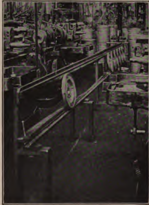
North End of Fly-Wheel Roll-Way Showing the commercial bar steel construction
