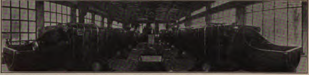
Power House, with 5,000 Horse-Power Gas Engine
