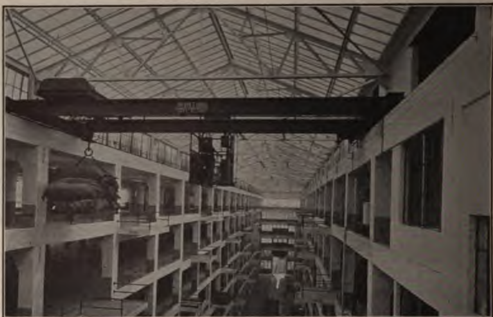
Looking East along the South Craneway, Showing Crane with Load
