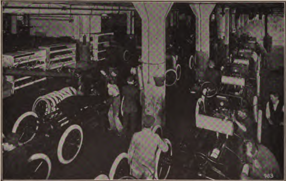
Applying Wheels to Chassis Looking northward from radiator platform
