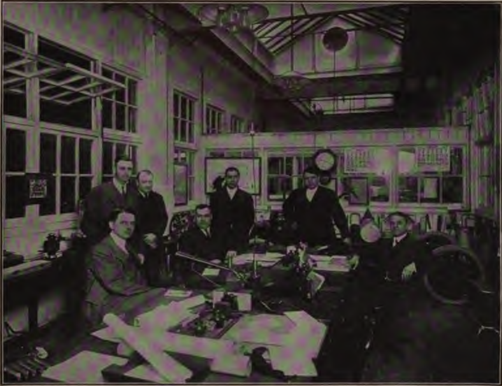
Interior of Machine-Shop Superintendent's Office and Group of the Principal Officials of the Machine Shop
