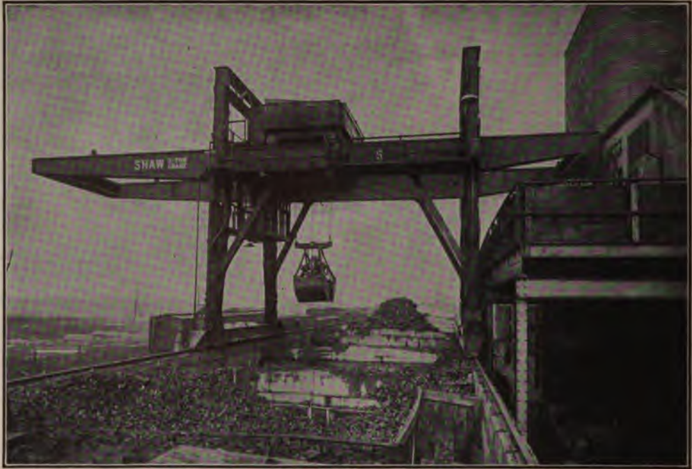
5-Ton Shaw Gantry Crane Covering the Sand, Coke and Scrap Bins on the North Side of the Ford Foundry
