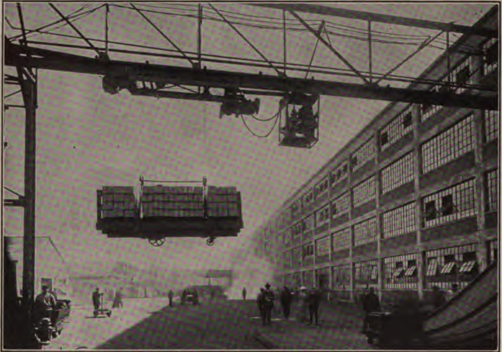
Monorail Trolley Hauling a Truck from Railroad Platform to Factory
