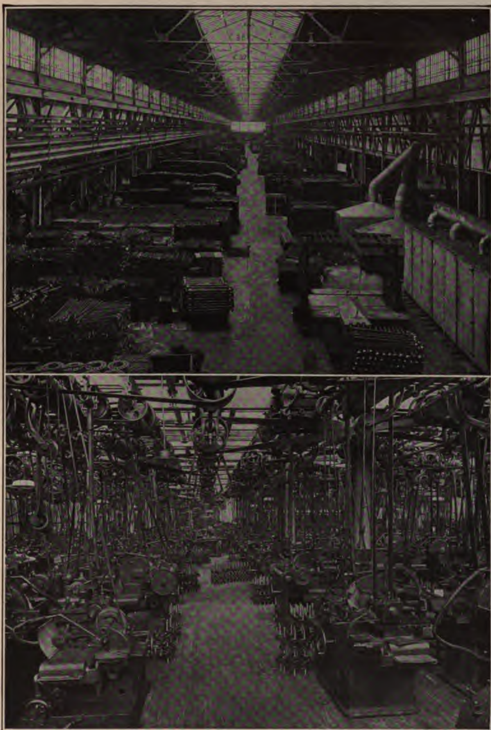
Above: A View Looking North Through the Main Craneway, Showing the Careful Manner in Which Stock is Piled. Note Light and Cleanliness of Shop. Below: General View Showing Close Machine Grouping
