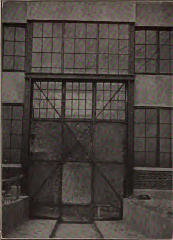
Craneway Door in East End of New Buildings Looking West
