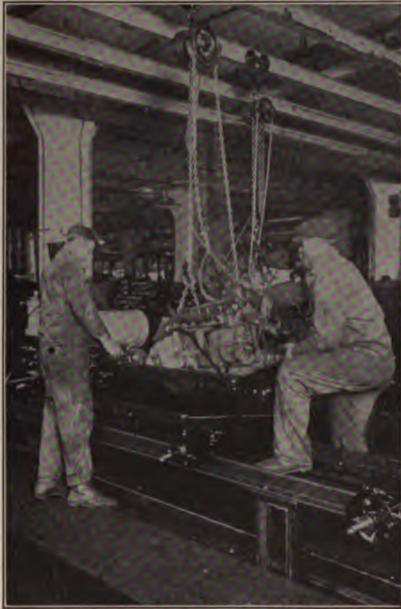
Lowering Motor to Place on Chassis Looking to southwest; shows overhead chain-hoist rails
