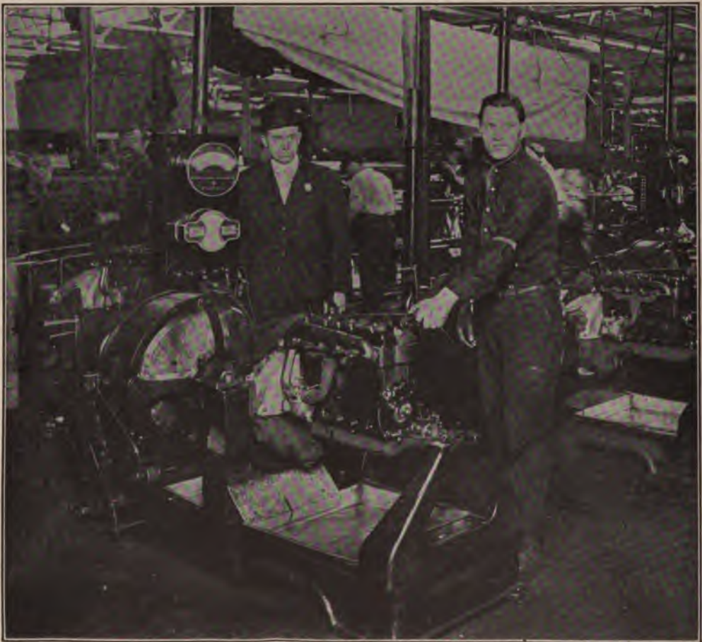
Single Motor-Testing Block, with Motor in Place for Running in
