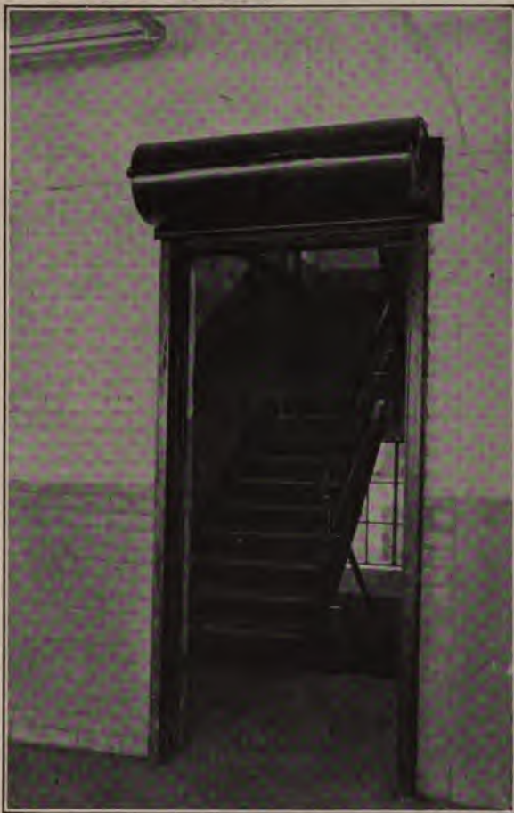
Stairway Next to the Elevator Shaft
