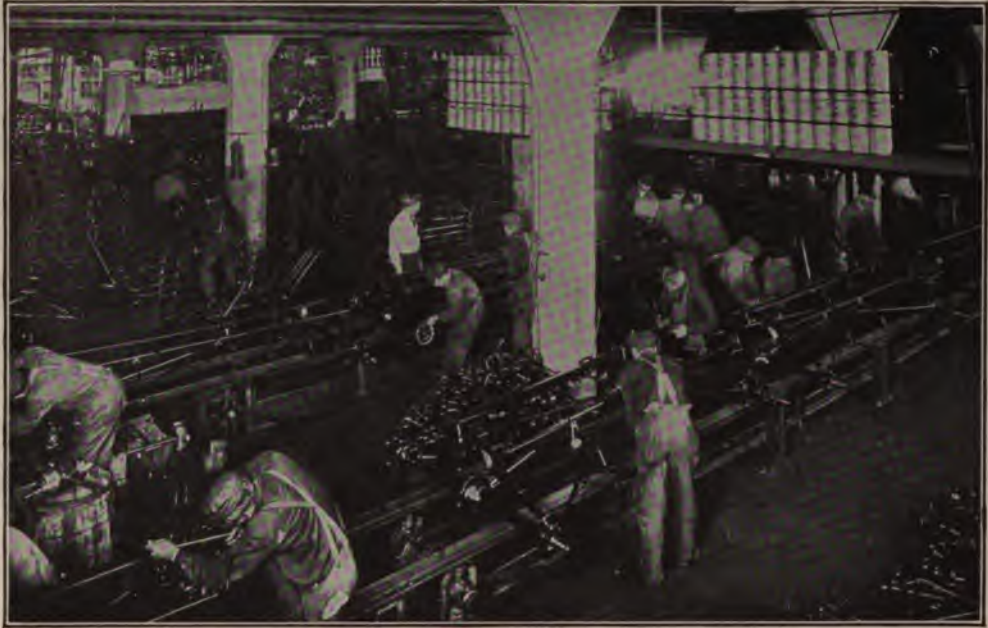
Placing Axles under the Chassis Frames and Springs
