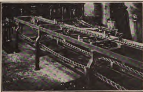
Idler End (West End) of Front-Axle Assembling Line
