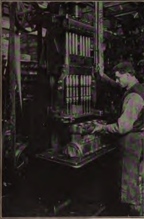
Operation 14—Finish Valve Seats on Foote-Burt 8-Spindle Drilling Machine
