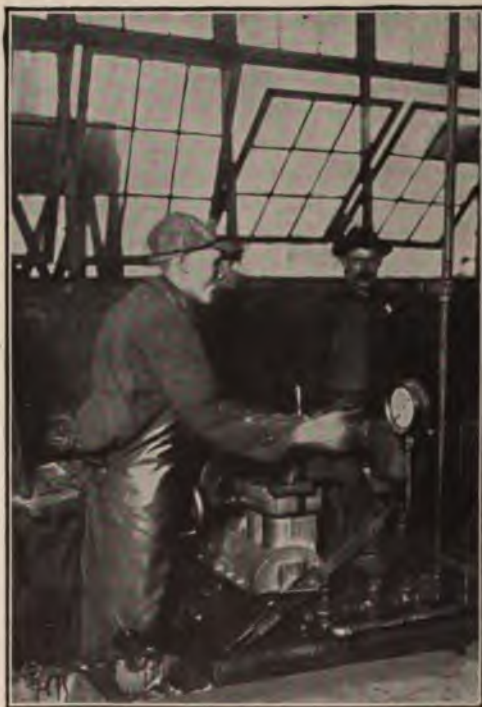
Cleaning Cylinders Hydraulic test for leaks
