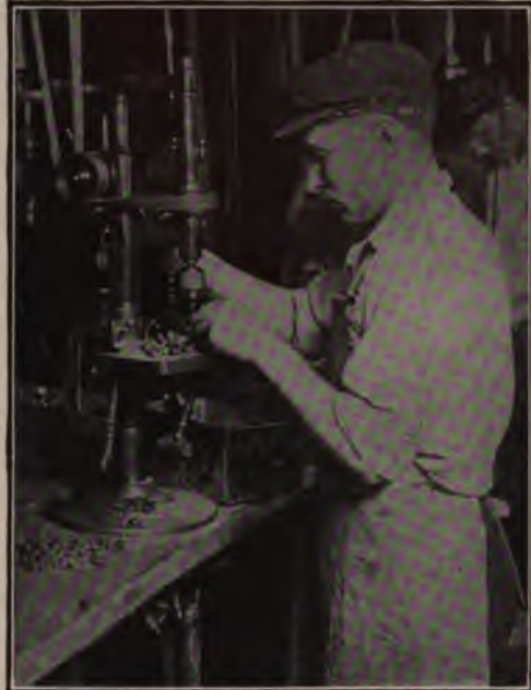
Operation 7 on Roller-Clevis Brass Casting, T-672
