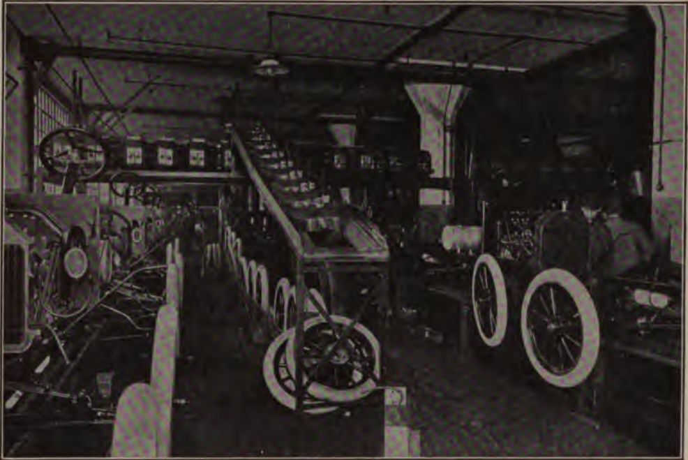
Applying Radiator to Chassis Looking southward, showing radiator platform
