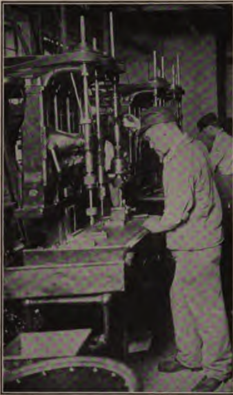
Operation No. 2. on T-4446. Drilling Two Holes
