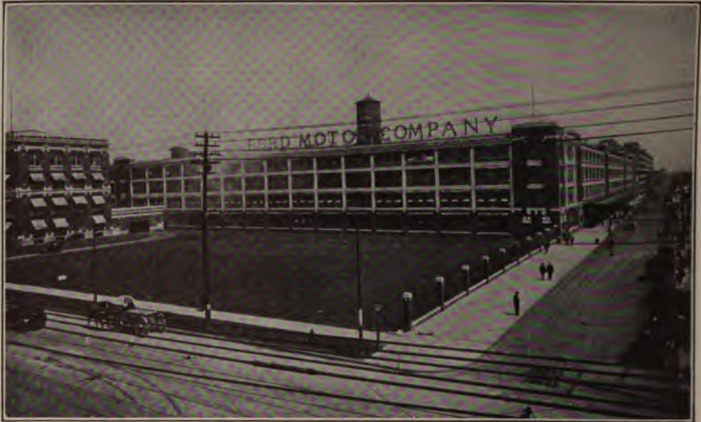
Manchester Avenue Side of the Ford Plant, Looking Northeast from Woodward Avenue
