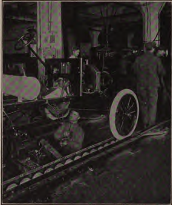
Workman in Pit under Chassis, Capping Front-Axle-Brace Globe
