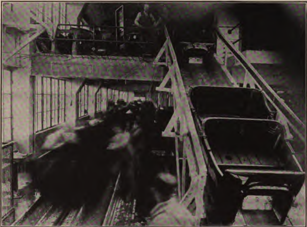
Looking South along the "Rubbing Deck"
