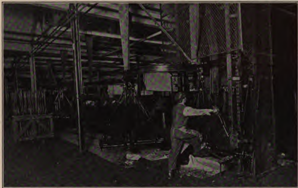
Putting the Rear-Axle Assembly into the Elevator Carrying It to the Floor Above
