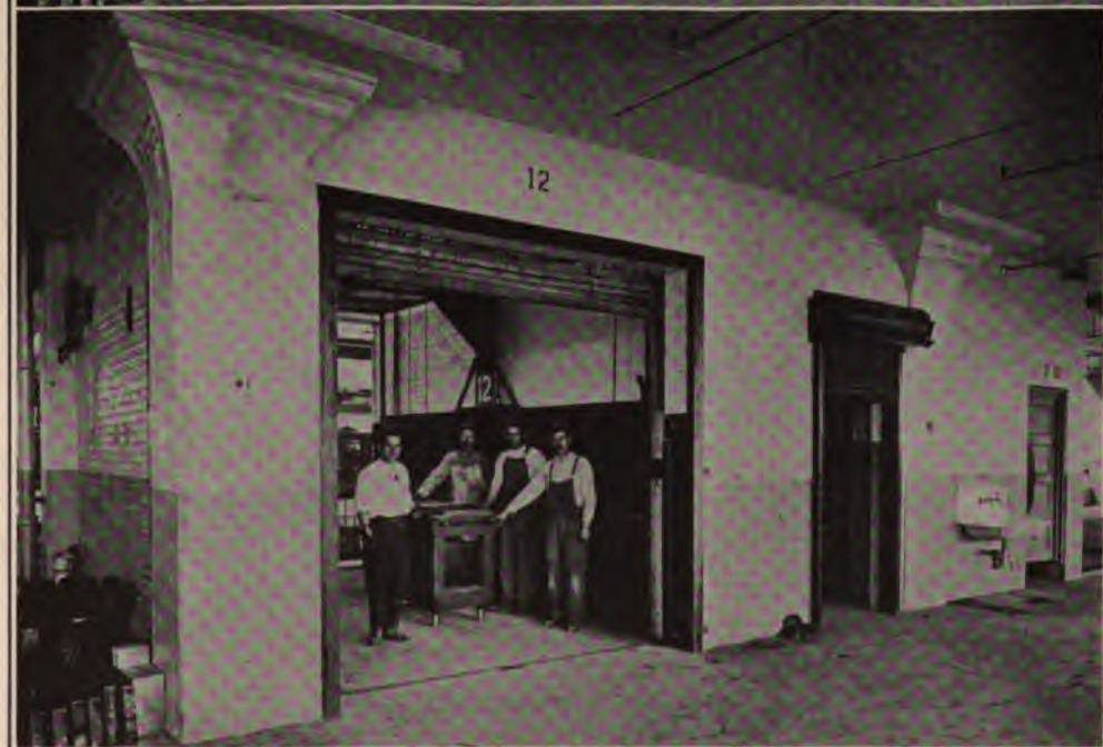
Elevator-Shaft Door, South Building, with Gate Down and with Gate Raised
