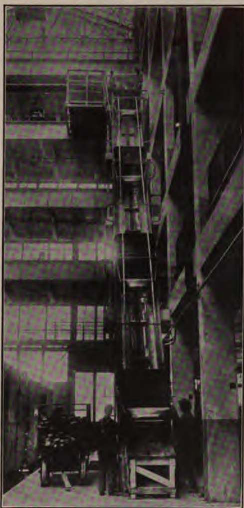
The Conveyer Carrying the Rough Unfinished Bodies from the Unloading Dock to the Fifth Floor
