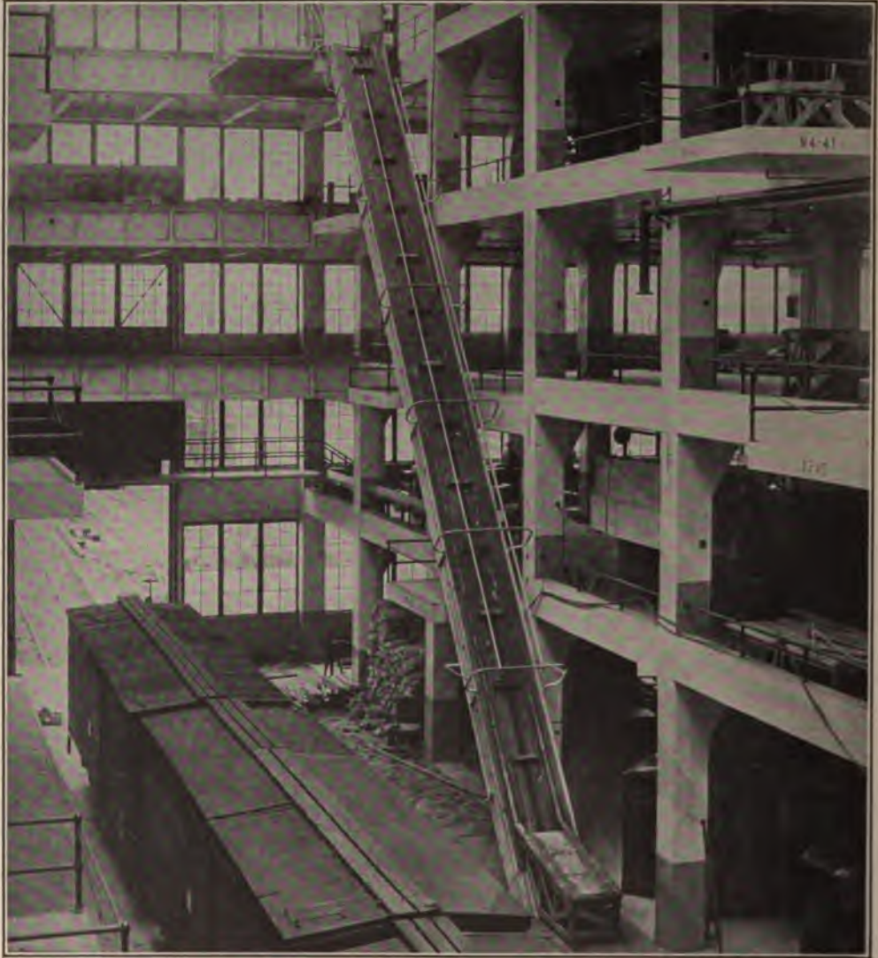
Body Elevator East End of South Craneway, Showing Railway Track Door Lifted
