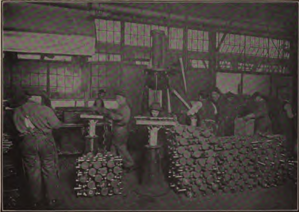
In the Heat-Treat Shop. Rough-Straightening Crank-Shafts
