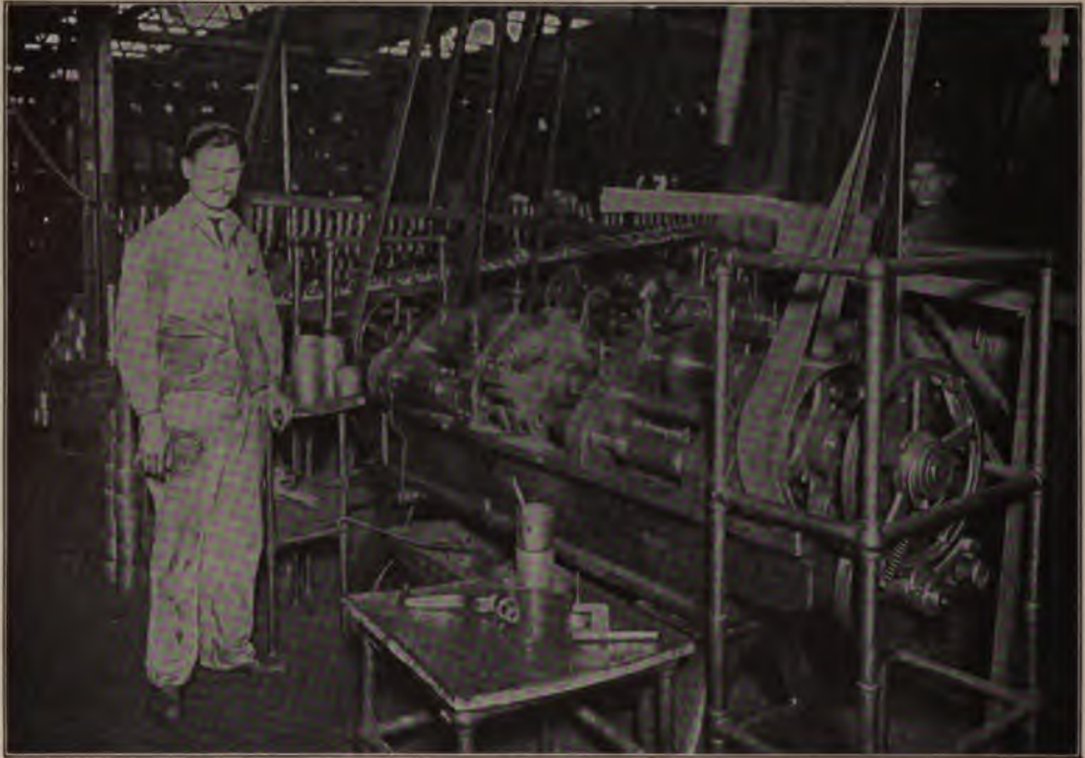
Finishing Pin Holes in Pistons
