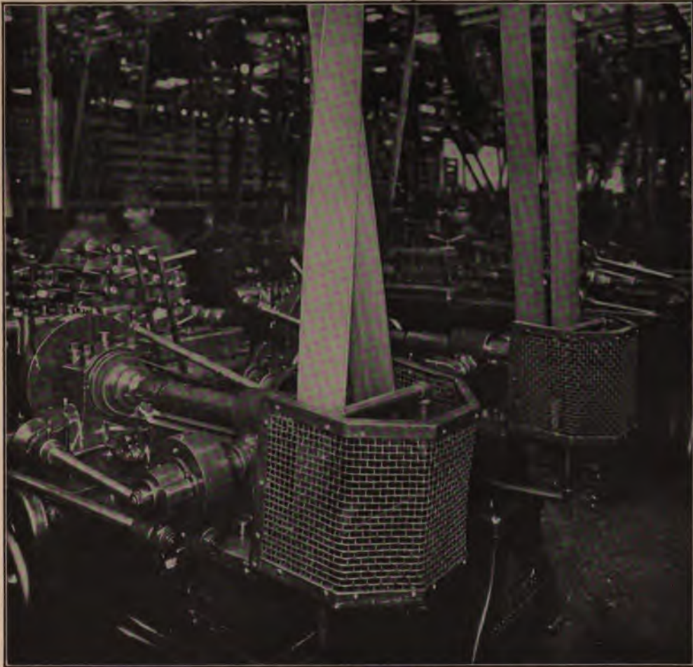
Wire Cage around Belts in Machine Shop
