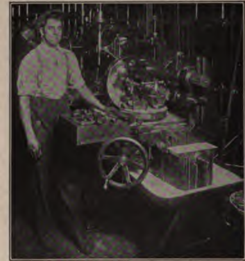
Milling the Fork-Lugs of Component T-248
