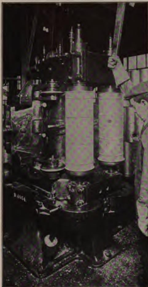
Rolling in Ends of Gasoline Tanks
