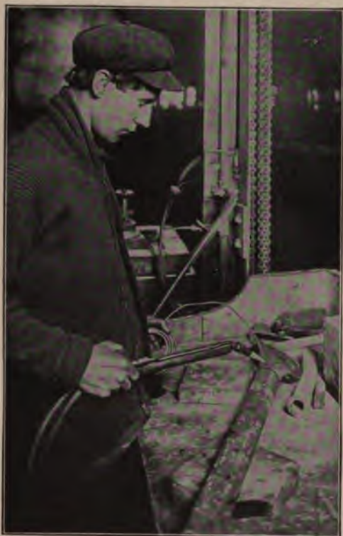
Spot-Brazing with Oxygen Torch
