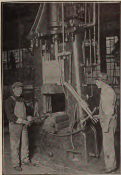
Re-Striking a Crank-Shaft
