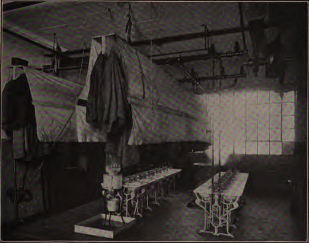
A departmental lavatory, with individual basins, water bottle, and canvas-covered coat hangers raised by rope and pulleys
