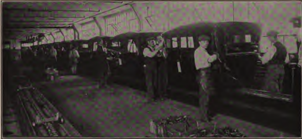
Fitting Top on Body, on Chain-Driven Line
