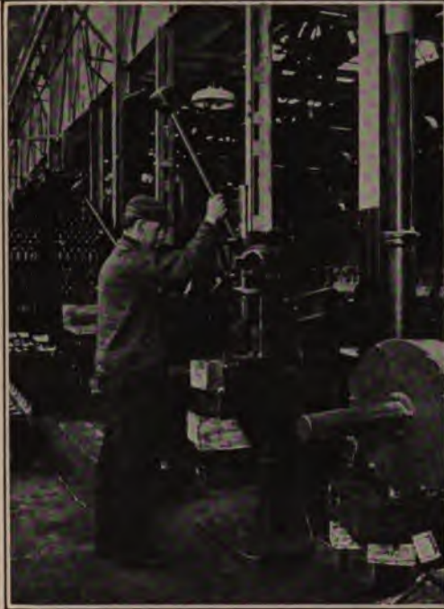
Safety Pad on End of Press Lever
