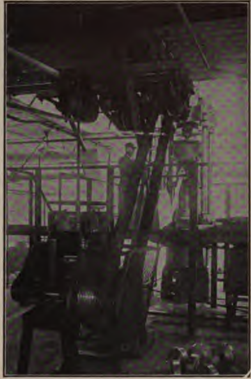
Forming Solder Ribbon on the Solder-Making Machine
