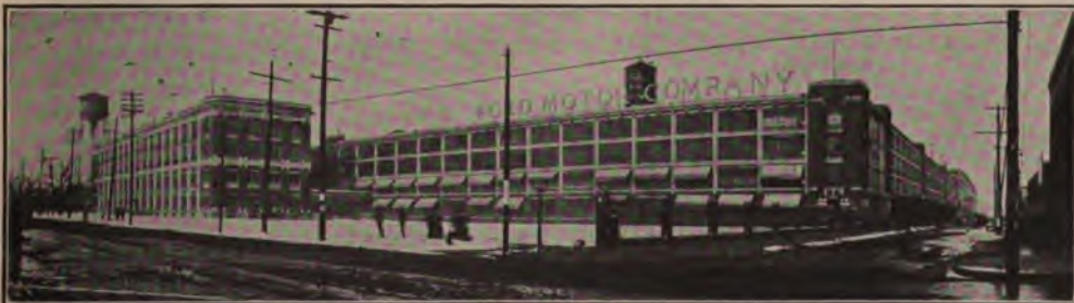
The Highland Park Plant, from the Corner of Woodward Ave. and Manchester St. The new buildings may be faintly seen down Manchester Street, which is at the right of the picture
