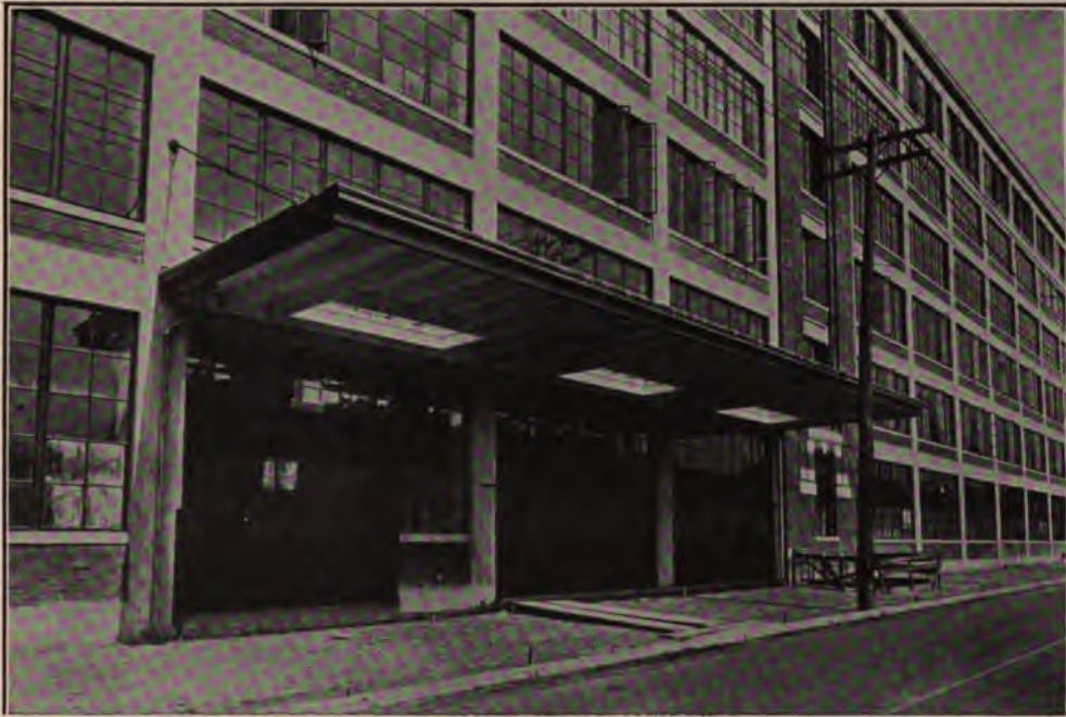
Doors on Manchester Avenue with Skylight Canopy Above
