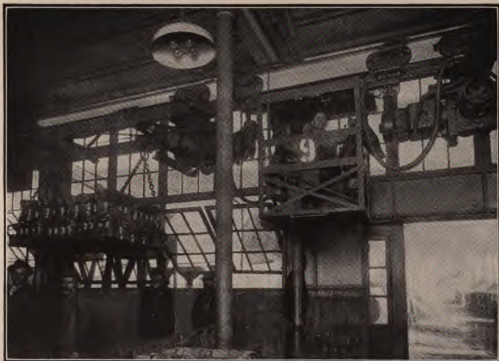
Cylinders Cleaning Floor. Monorail for Transporting Cylinders to Machine Shop
