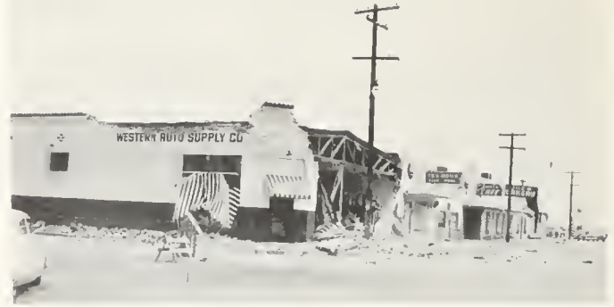
FIGURE 4. Brick construction on alluvium. Damaged building in business district of Arvin. Other buildings, of reinforced concrete, were undamaged.
