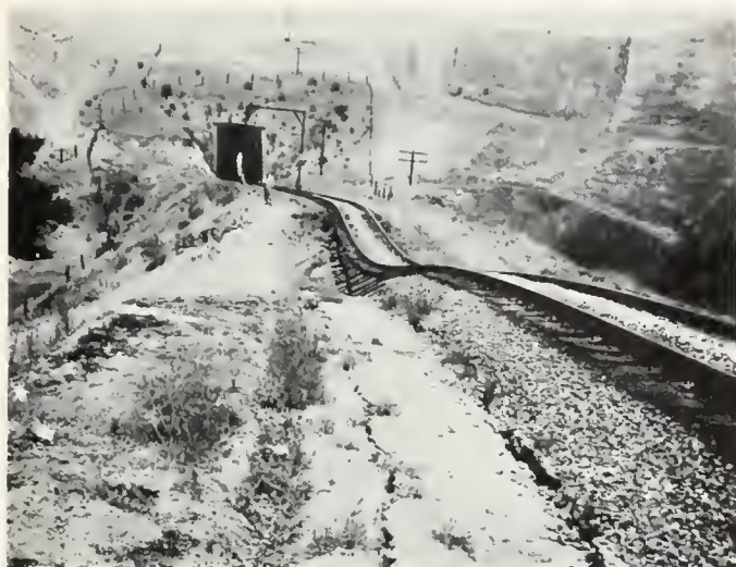
FIGURE 5. Track east of Tunnel 1, from south side of track.
