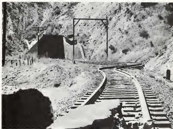
FIGURE 8. View east from east end of Tunnel 3; Tunnel 4 in background.
