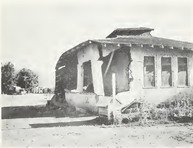
FIGURE 11. Detail of damaged schoolhouse shown in figure 10.
