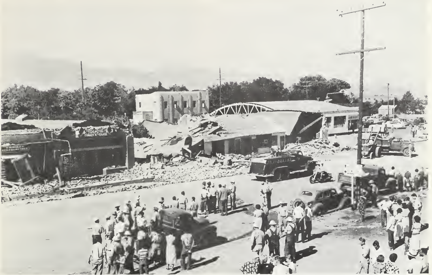
FIGURE 3. Looking southwest across Main Street, Tehachapi; undamaged reinforced concrete building, left center. Wide World Photos.
