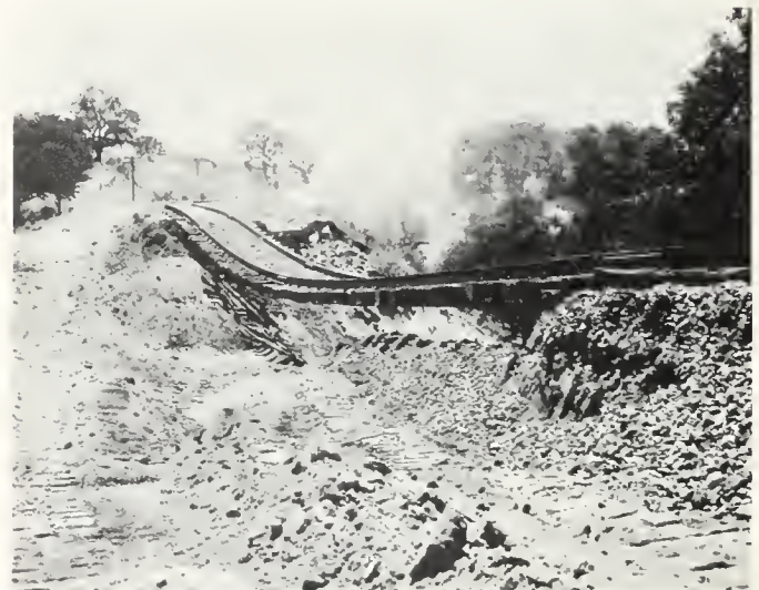
FIGURE 4. Track east of Tunnel 1. View west from north side of track.
