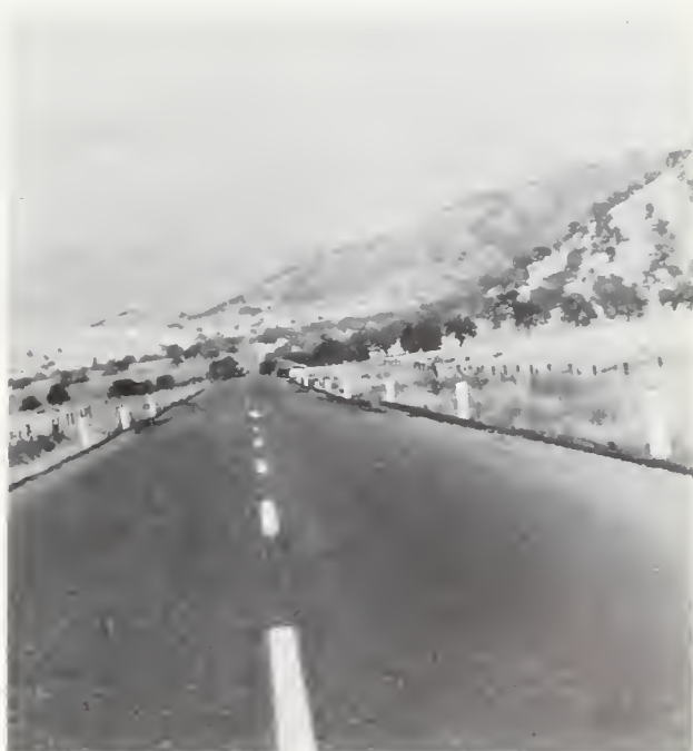
FIGURE 3. Horizontal displacement of highway shown by center line. View east on Highway 466. Not on trace of White Wolf fault.
