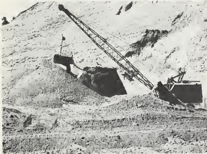
FIGURE 14. Dragline working at west portal of Tunnel 4, August 3, 1952.
