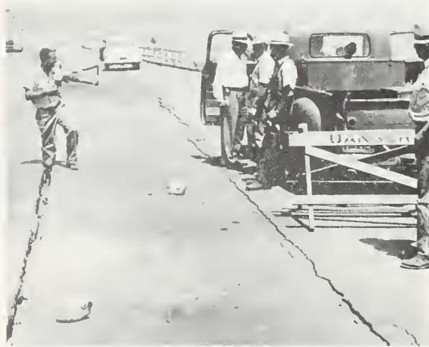
FIGURE 13. Longitudinal cracking in pavement of northbound lane of U. S. Highway 99 near Grapevine. This type of cracking took place in filled sections where adjacent concrete slabs were not held together with tie bolts.
