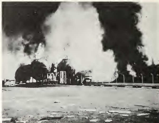
FIGURE 4. A mass of butane which escaped from these 2500-barrel spheres became ignited by an electrical spark, causing the initial explosion and resultant fire at the Paloma cycling plant.
