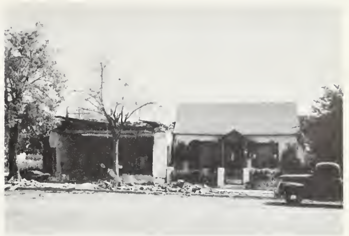
FIGURE 16. Frame construction on alluvium. Undamaged building in Tehachapi. Adjacent adobe structure was extensively damaged.
