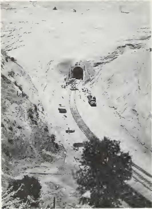
FIGURE 9. Looking west toward Tunnel 3 from position above Tunnel 4.
