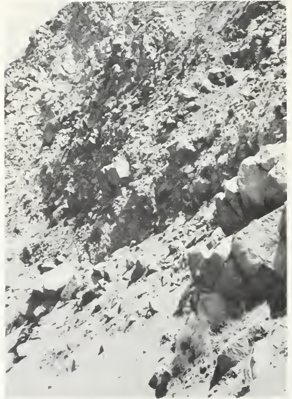
FIGURE 26. Natural hill slope above rock slides on highway in Kern Canyon, showing loose and fragmented granitic rock.
