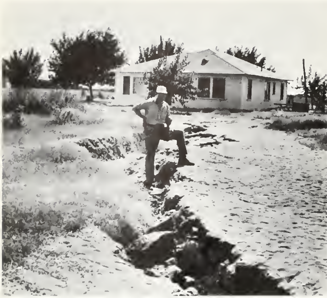
FIGURE 8. View west toward Jones ranch house, showing cracks in alluvium. These cracks are not parallel to the fault trace but are in an area of extensive lurch cracking on the valley floor. At Edison Road about 4 miles southwest of Arvin. Photo by Lawrence W. Chasteen.
