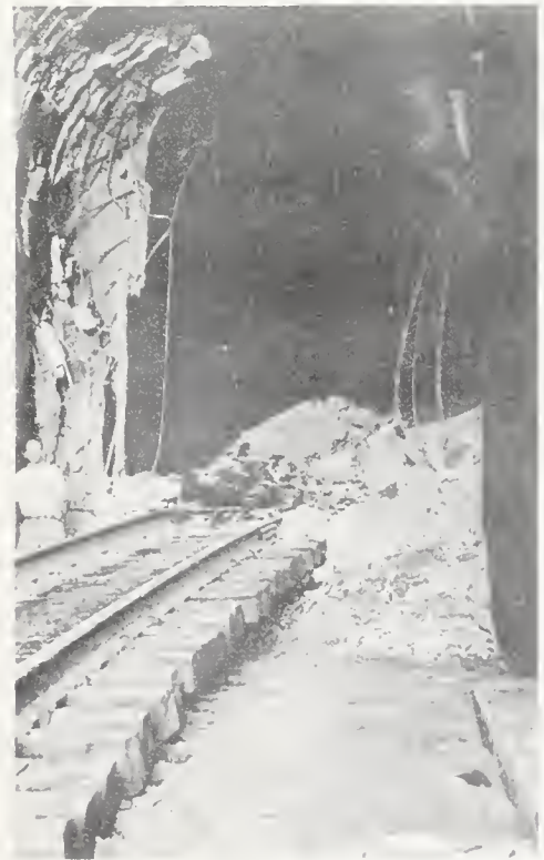
FIGURE 7. View in tunnel 4. Normal fault dipping 72° toward the camera has offset the walls and lifted the track 3 feet. The slender curved rods are steel reinforcement.
