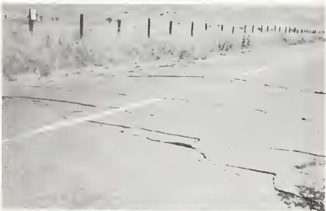
FIGURE 5. En echelon cracks in Arvin road at point 28, indicating left lateral movement.
