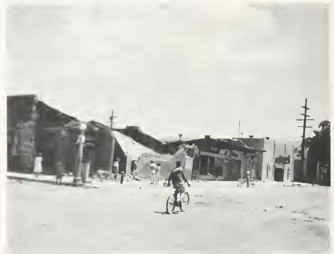
FIGURE 5. Brick construction on alluvium. Damaged buildings in business district of Tehachapi. Much damage caused by roof falling into building when brick walls collapsed. Undamaged reinforced-concrete theater building at right.
