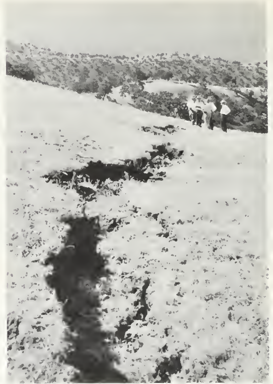
FIGURE 20. Crack in hill on ridge between Caliente and Tehachapi Creeks. Elevation 3000 feet. President Russe's inspection party, Southern Pacific Company, in background.
