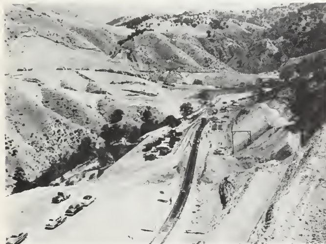
FIGURE 15. Looking east from position above west end of old Tunnel 4, toward new fill, August 12, 1952.
