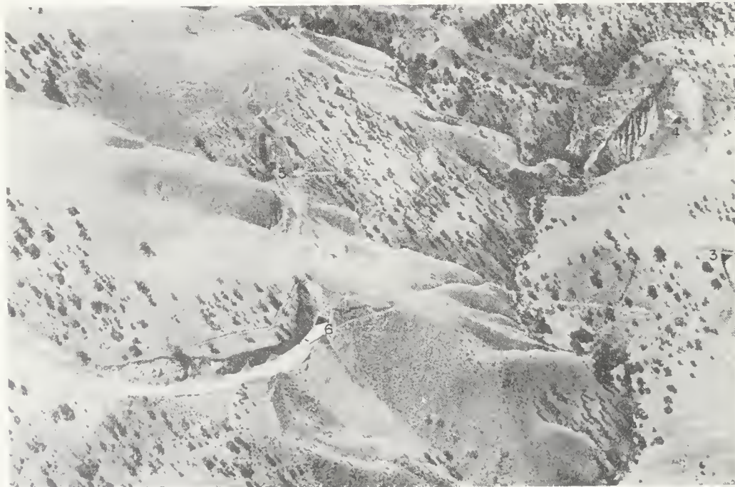
FIGURE 4. Air view of the S-curve in the Southern Pacific Railroad tracks east of Bealville, California. View south. The main valley separates tunnels 3 and 4 on the extreme right side from tunnels 5 and 6 left of center. Portal of tunnel 6 is distorted. Photo by John Shelton.
