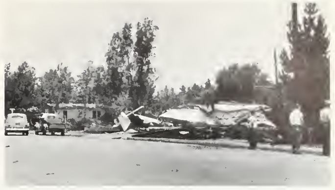
FIGURE 4. Elevated water tank that collapsed during July 21, 1952, earthquake. Third and A streets, Bakersfield. Photo by Gordon B. Oakeshott.
