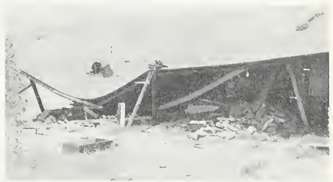
FIGURE 8. Grapevine Motel, U. S. Highway 99. Photo courtesy Chief, Seismological Field Survey, U. S. Coast & Geodetic Survey.
