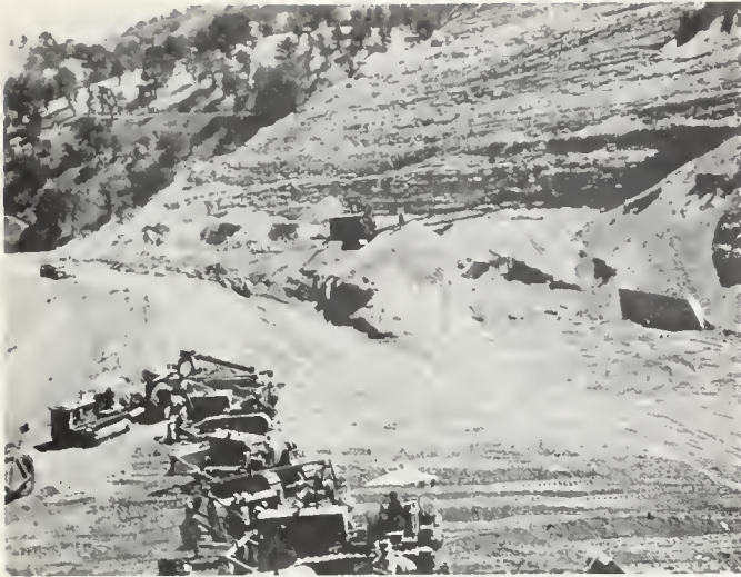
FIGURE 13. Work in progress between Tunnels 3 and 4, August 1, 1952.
