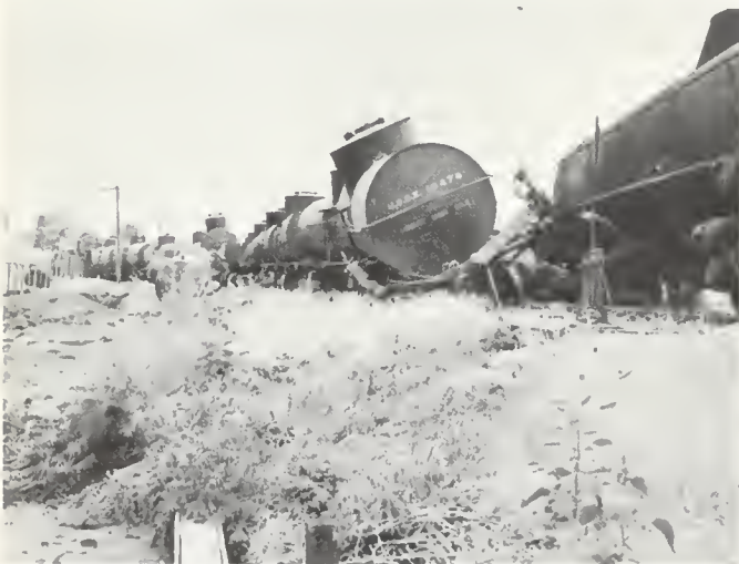
FIGURE 3. Tank cars overturned on Oil City Branch by earthquake.
