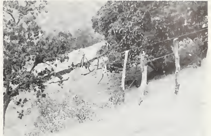
FIGURE 3. Stretched fence at point 20; tensional trace in middle ground.
