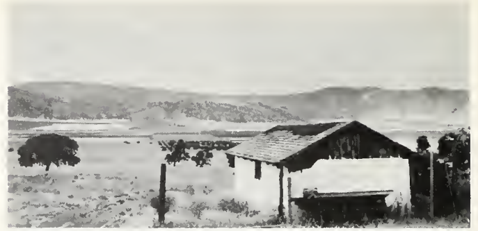
FIGURE 13. Adobe construction on a few inches of fill overlying rock. Undamaged building on south side of Cummings Valley.
