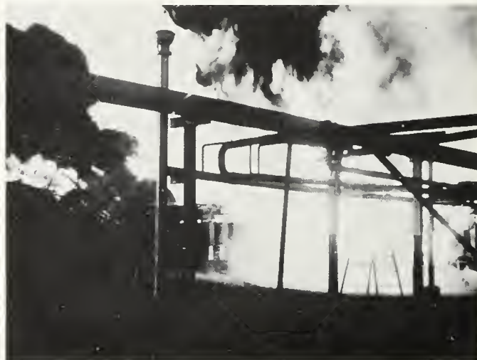
FIGURE 5. A closeup of the fiercely blazing skeletal remnants of one of the large cooling towers. A gigantic blowtorch effect was caused by the ignited gases which are normally being cooled beneath the towers.
