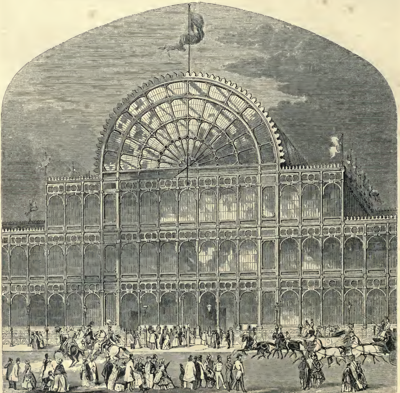
SOUTHERN ENTRANCE TO THE TRANSEPT.
